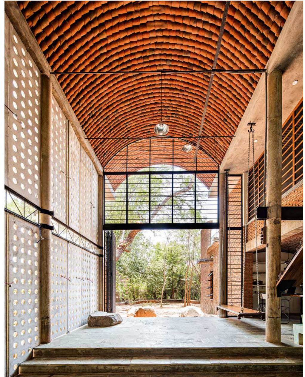
Figure 9, Anupama Kundoo, 2000. Wall House vaulted ceiling made of stacked terracotta pots. [Photograph]
