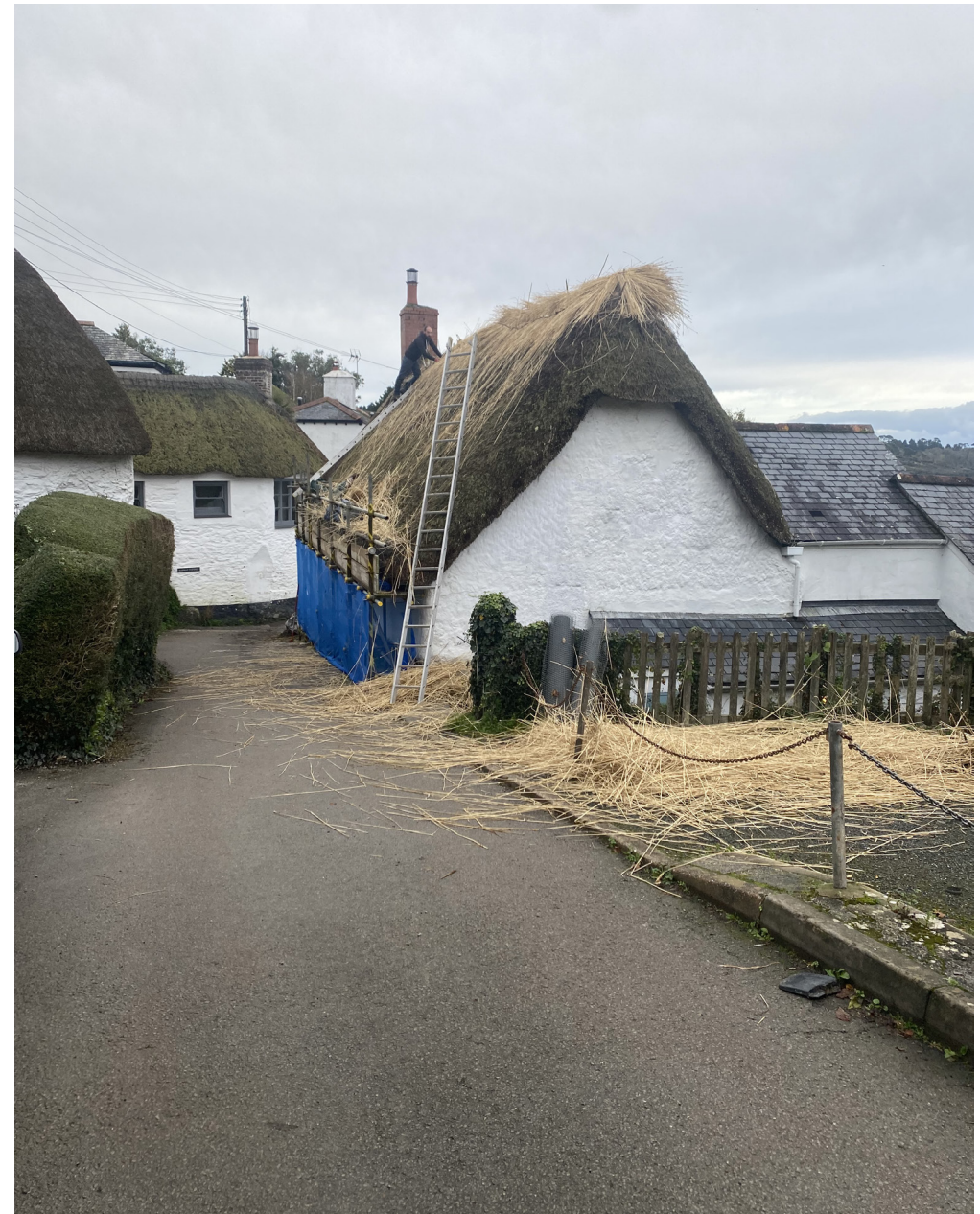
Figure 3, Author's Photograph 2021. Vernacular Roof Repair in Helford, Cornwall. [Photograph]
